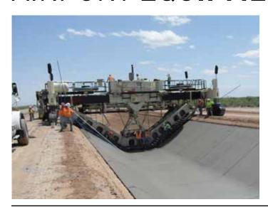
As an alternative to a custom built solution, G&Z's Highway and Airport Concrete Paving Equipment can be converted into canal and reservoir liners with minimal modification. The G&Z TC1500 can also be converted to a cure jumbo for canals and reservoirs.
